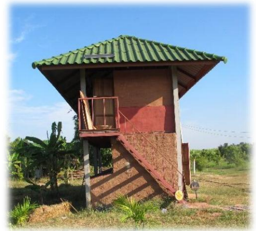
A compost toilet with a large chamber under the toilet
